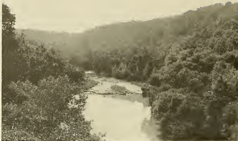
VIEW DOWNSTREAM FROM EDMONDSON BRIDGE. DICKIE DAM IN FOREGROUND.
